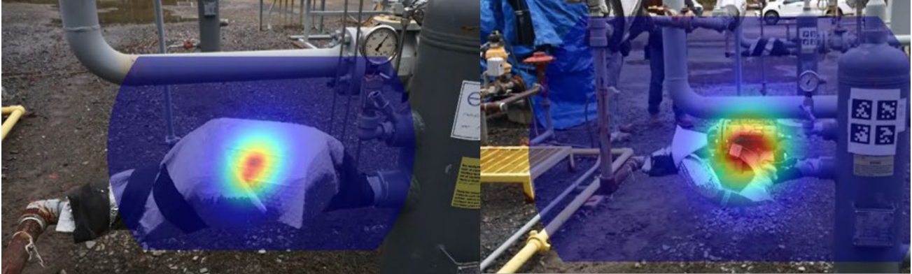
Figure 5. Emissions were detected under a bubble wrap, and the recording on the regulator after the wrap was removed.
